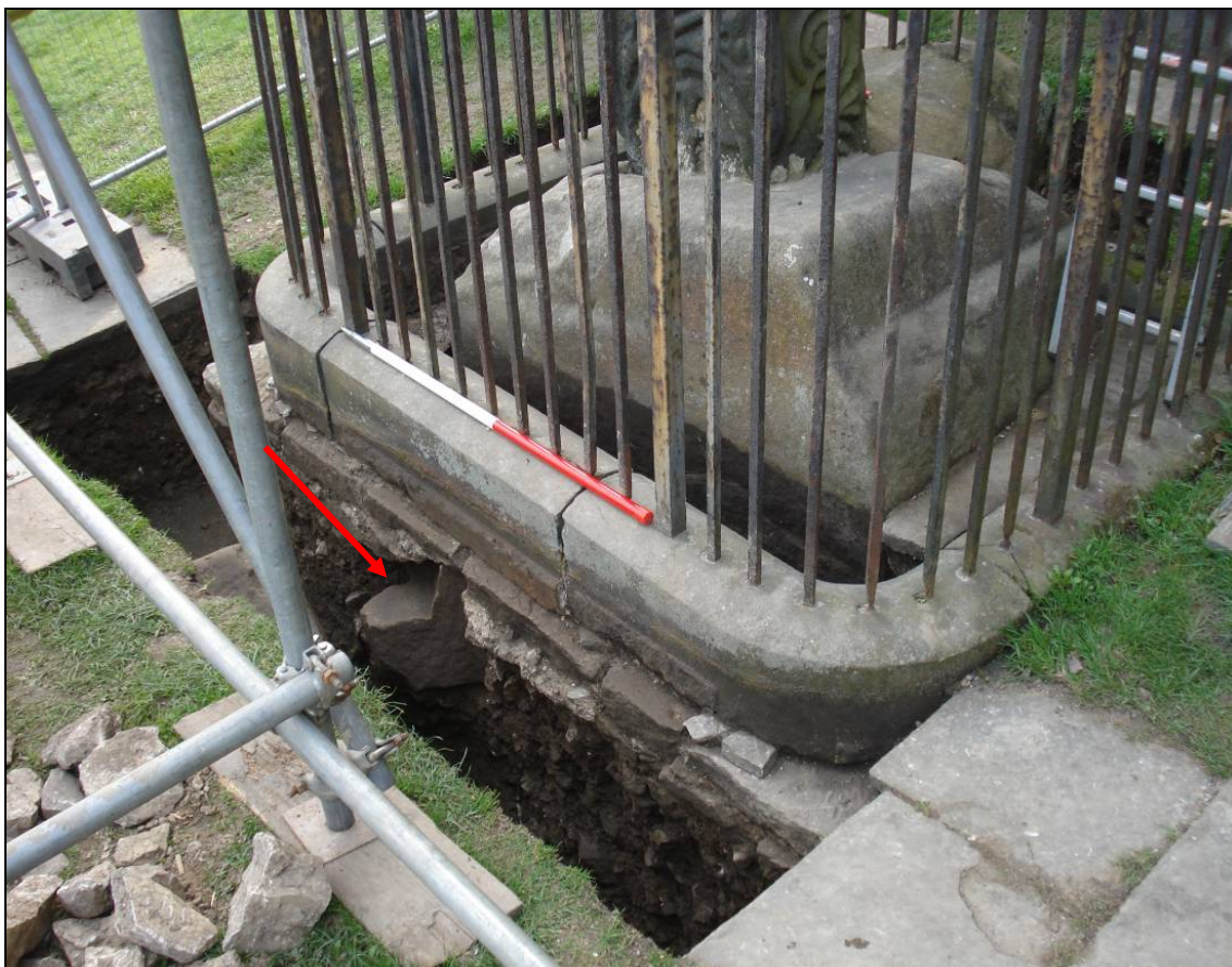
Figure 19: Architectural fragment within wall (211) projecting from the west facing section 3 (scale 1m)
