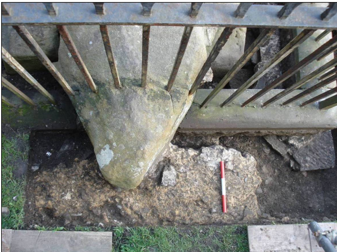
Figure 26: Chock stone overlying a mortar layer (210), looking east (scale 300mm)
