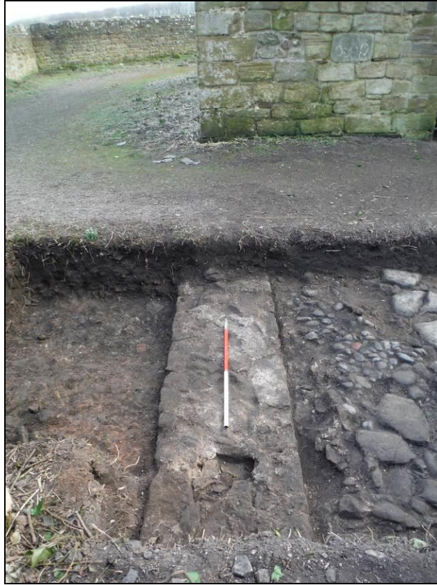
Figure 36. Sandstone wall foundation (1107), belonging the 18th century Mansion House, showing its alignment with the north-east wall of the pele tower (scale = 0.5m graduations).
