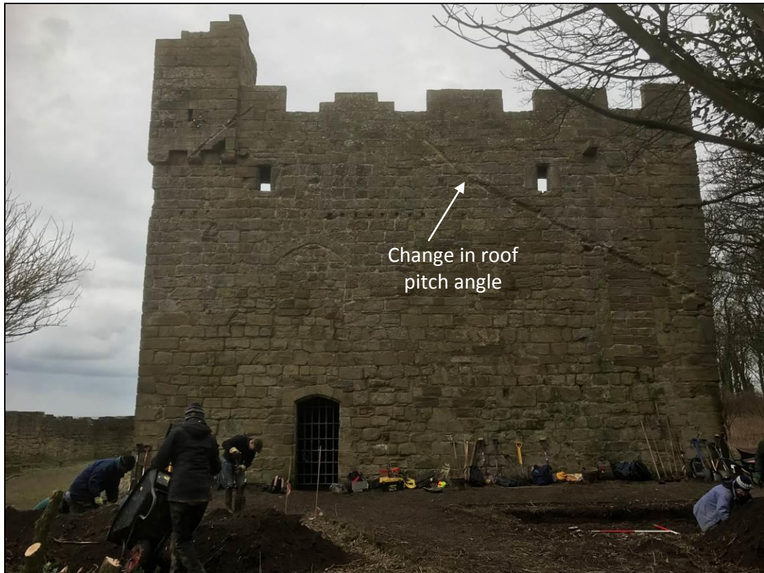
Figure 34. The north-west elevation wall of the pele tower showing the construction groove for the 18 th century mansion house pitched roof. Note where the pitch changes angle, demonstrating the two separate construction phases of the 18 th century mansion house.
