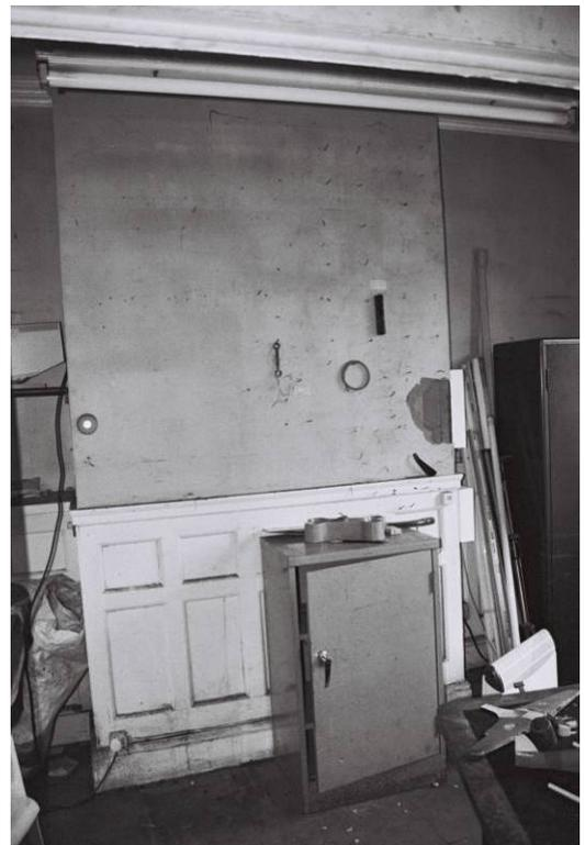
Figure 28: Fire place blocked with dado panelling
