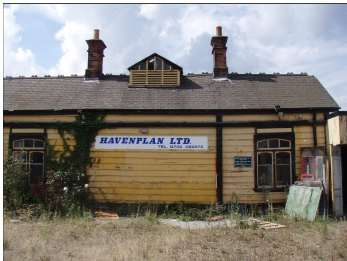
Figure 13: Northern end of the east elevation showing chimney stacks and louvre lantern
