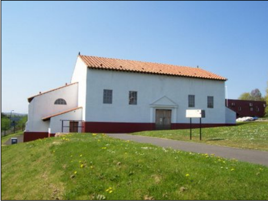
Figure 13. The full-size reconstructed Roman bath house at Wallsend Roman fort, North Tyneside.
