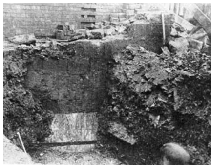
Figure 1. The basal courses of the bastion tower (reproduced from Armstrong’s 1930 report).
