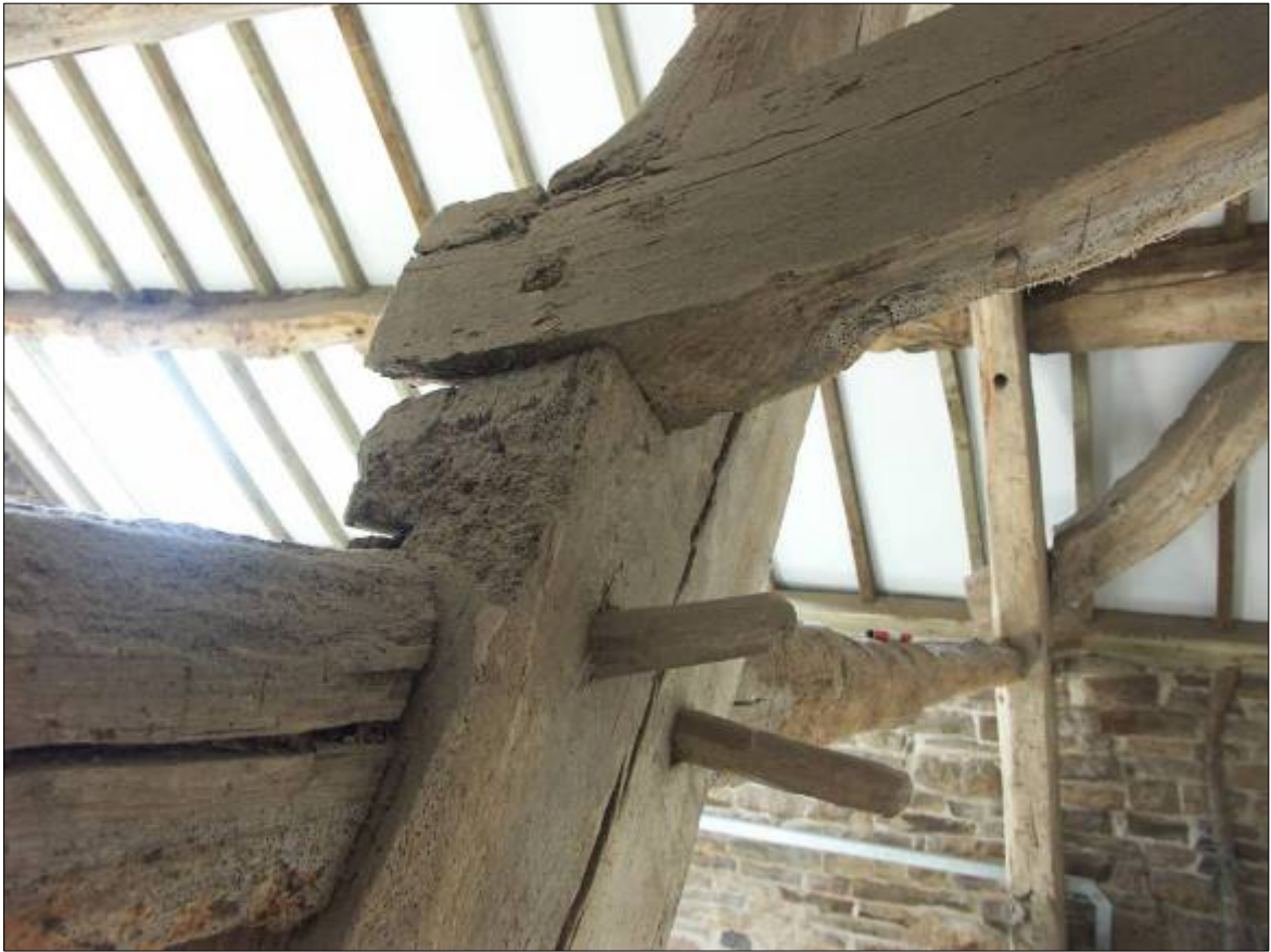
Plate 45. Detail of the halved joint for the tie-beam with tusk pegs.
