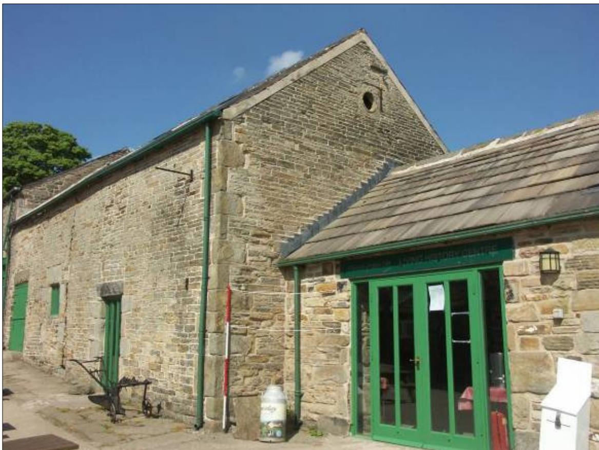
Plate 35. East elevation of Building I, showing round owl hole in the gable.
