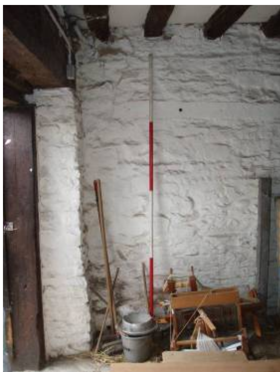
Plate 39. Interior of the western half of Building I showing the scar of a cruck blade in the south west corner.
