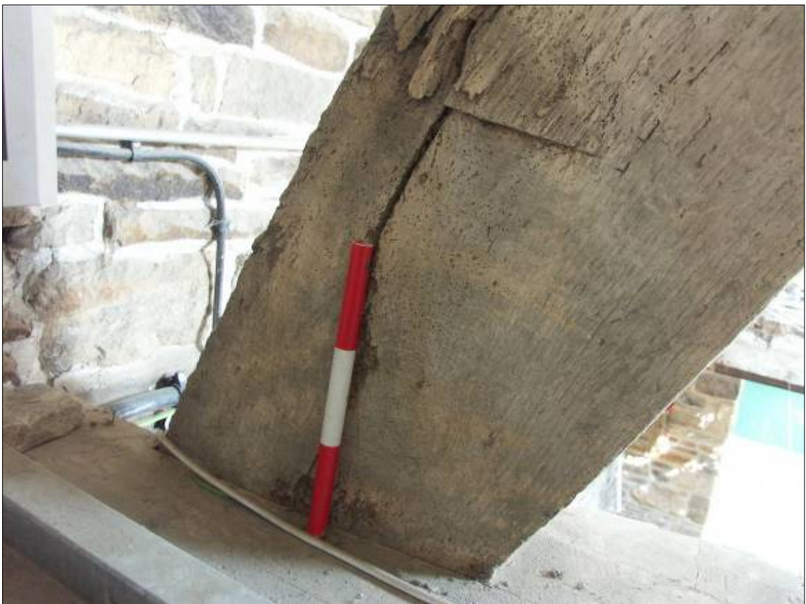
Plate 46. Pit-saw mark on the north blade of the cruck frame.
