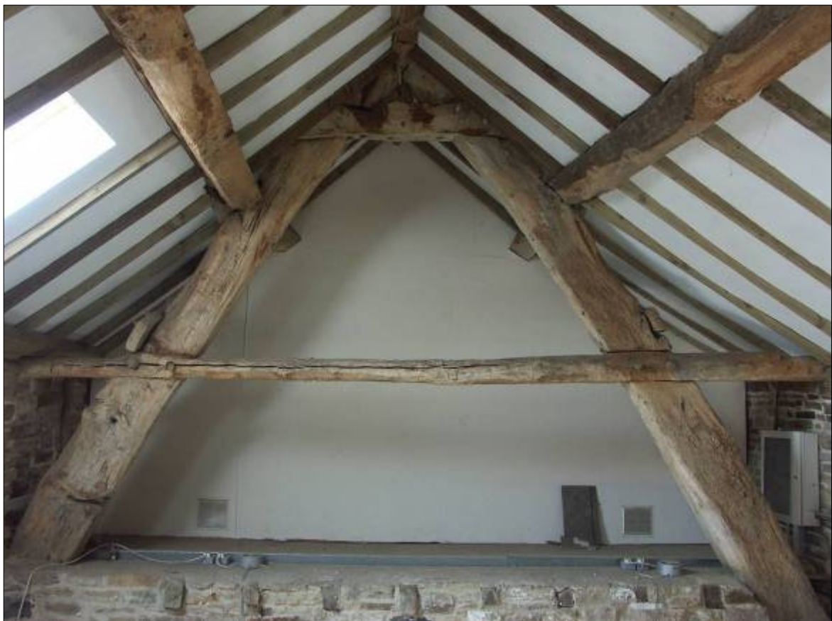
Plate 42. Detail of surviving cruck frame. Interior of Building I.
