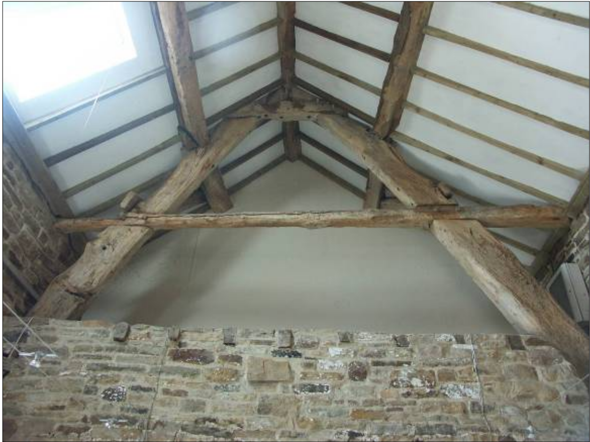
Plate 41. Interior of Building I facing west, showing surviving cruck blades, ridge beam, collar and tie beam encased in a later stone partition wall.
