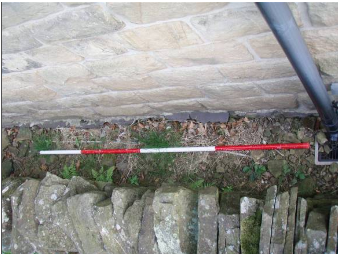
Plate 91. Detail of slate damp-proof course on the northwest wall of Building S.
