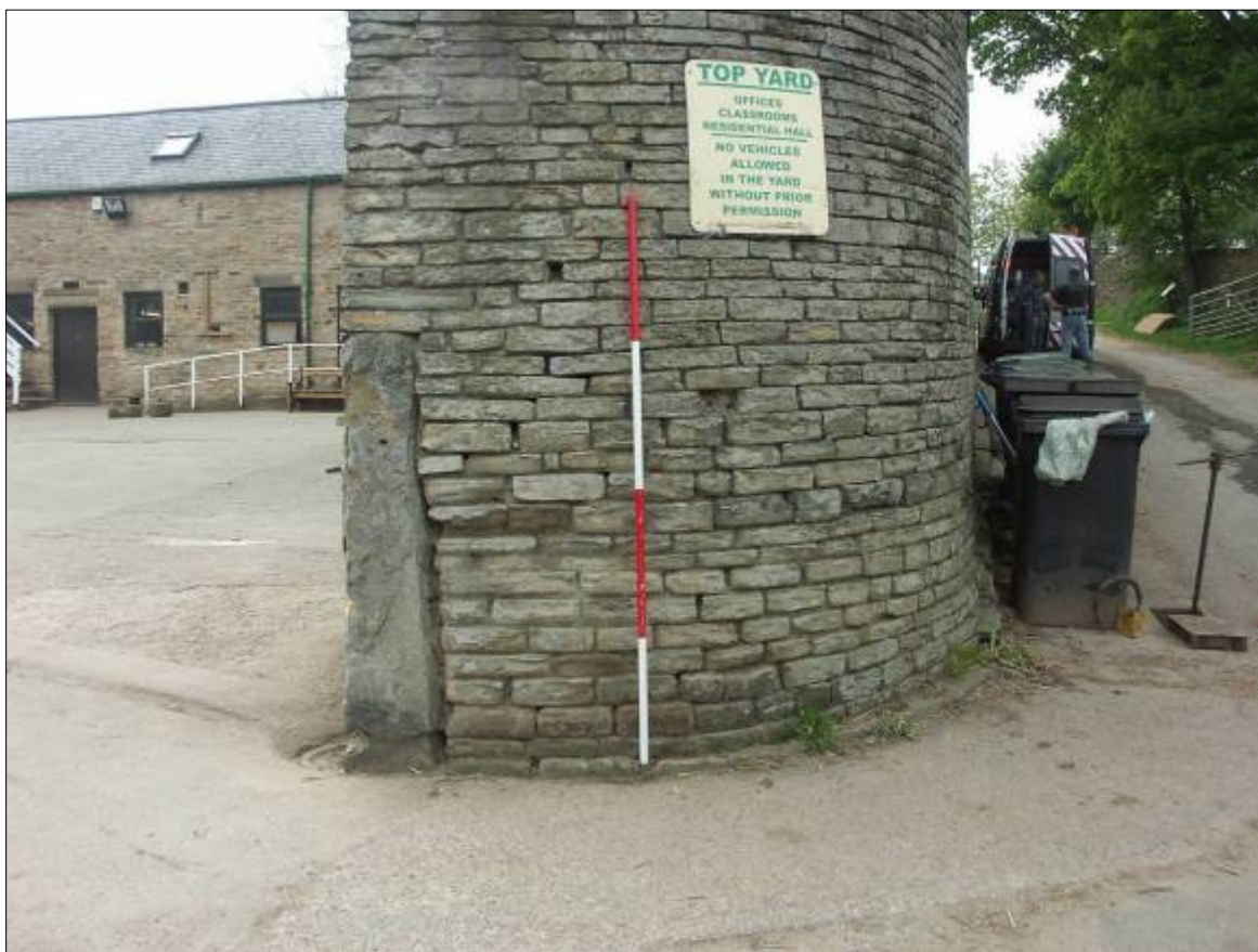
Plate 84. East elevation of Building Q showing walling built up over the gate-post.
