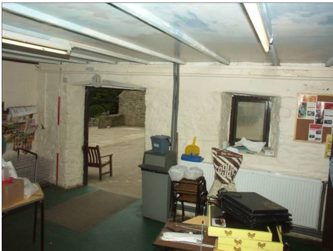
Plate 82. Ground floor of Building P facing south showing breeze-blocked partition wall on the left.
