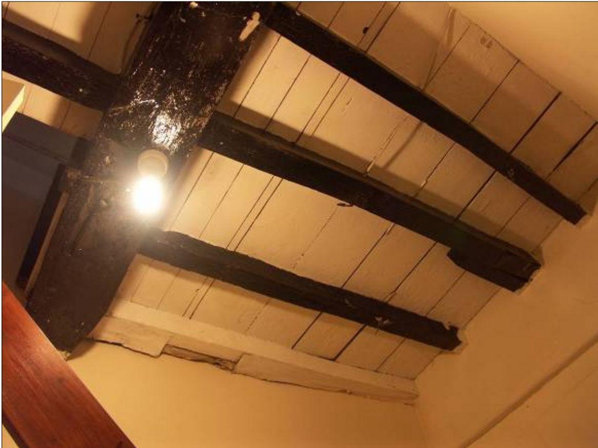
Plate 23. Ground floor of Building F. Interior showing original timber floor boards of the first floor.
