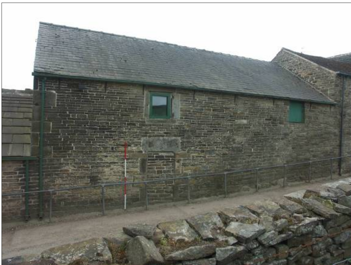
Plate 36. North elevation of Building I, showing crack associated with the location of a cruck frame.
