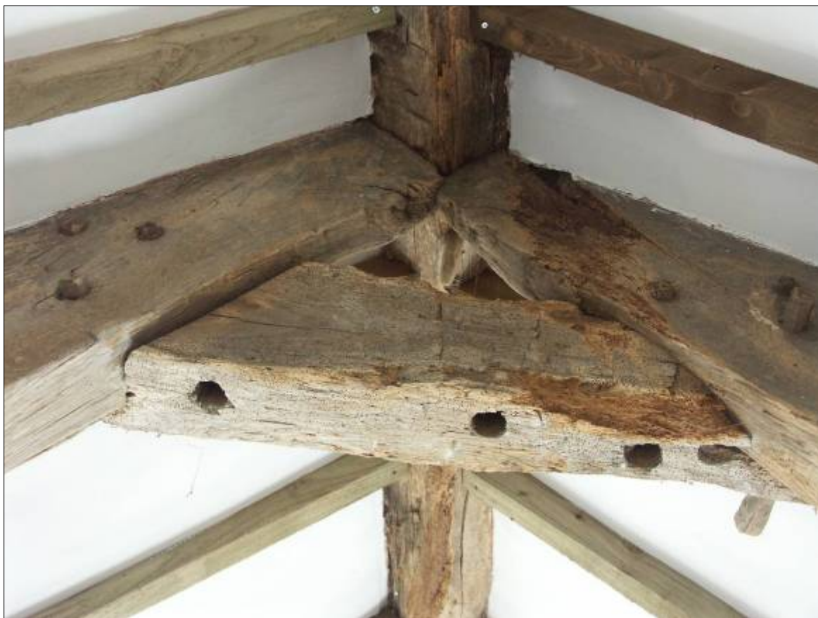
Plate 43. Detail of the apex arrangement of the surviving cruck frame.
