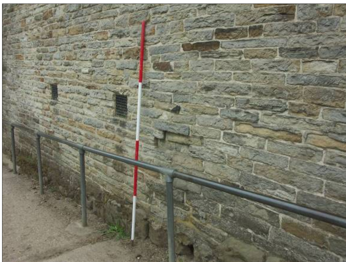
Plate 29. Detail of a possible scar associated with the location of a, now removed, cruck frame in the north wall of Building H.
