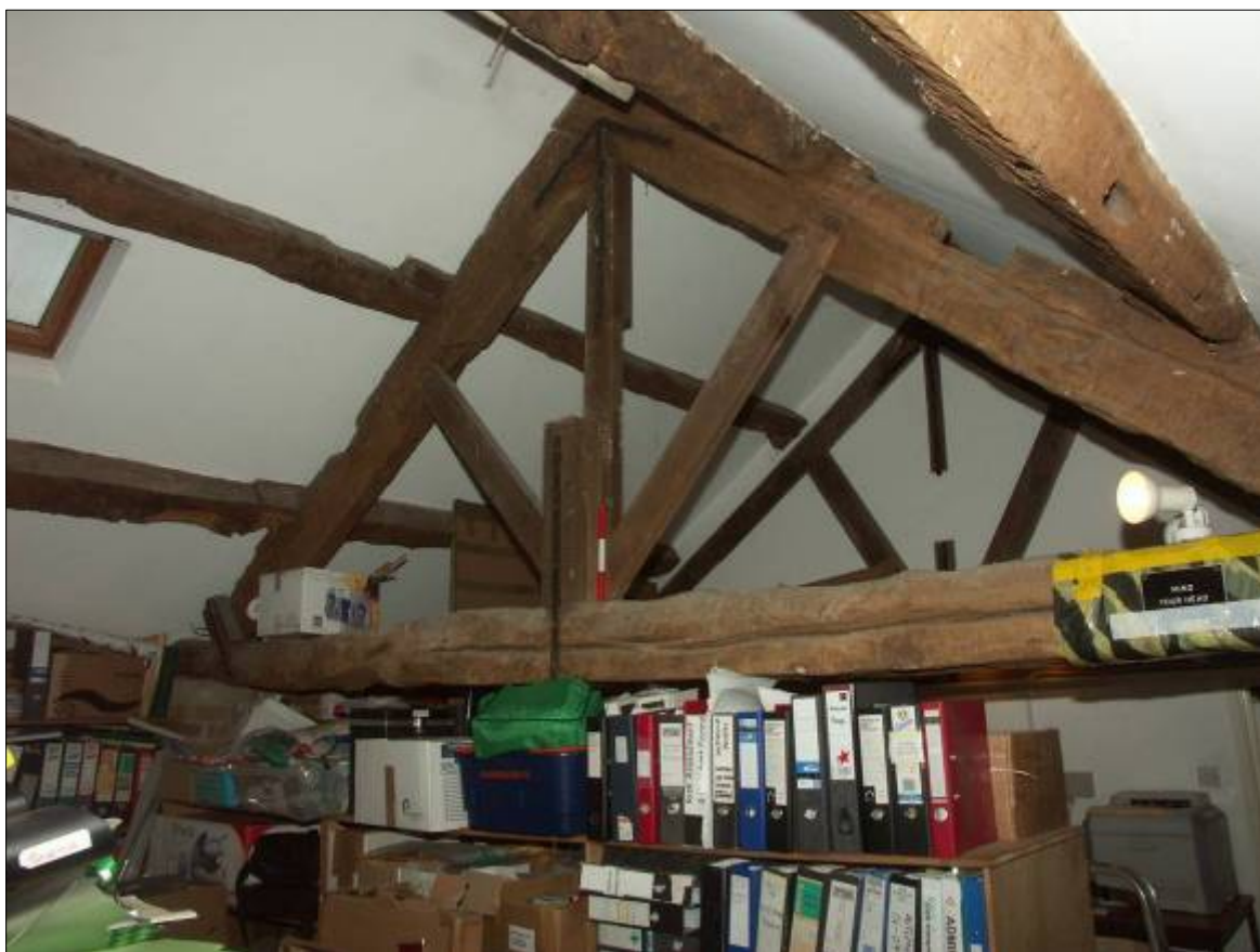
Plate 78. First floor of Building O facing south. Interior showing king post truss with remodelled side purlins.
