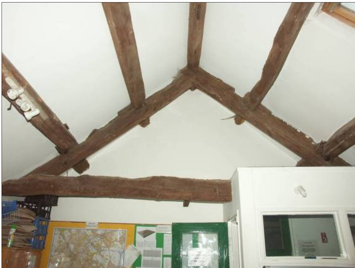
Plate 76. First floor of Building O facing north. Interior of first partition wall showing a couple-close truss.
