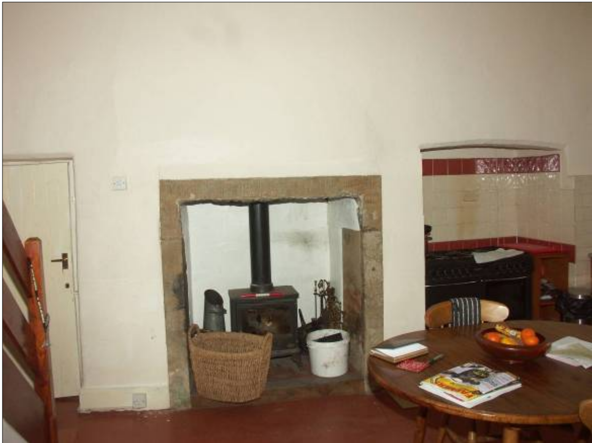
Plate 21. Ground floor of Building F. Interior of north wall showing modified central fireplace with original doorway on the left and possible built-in cupboard opening on the right.
