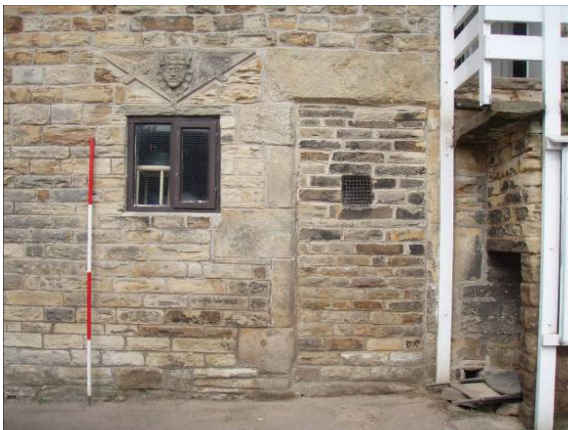
Plate 67. Blocked doorway and inserted stone carving on the east wall of Building O.
