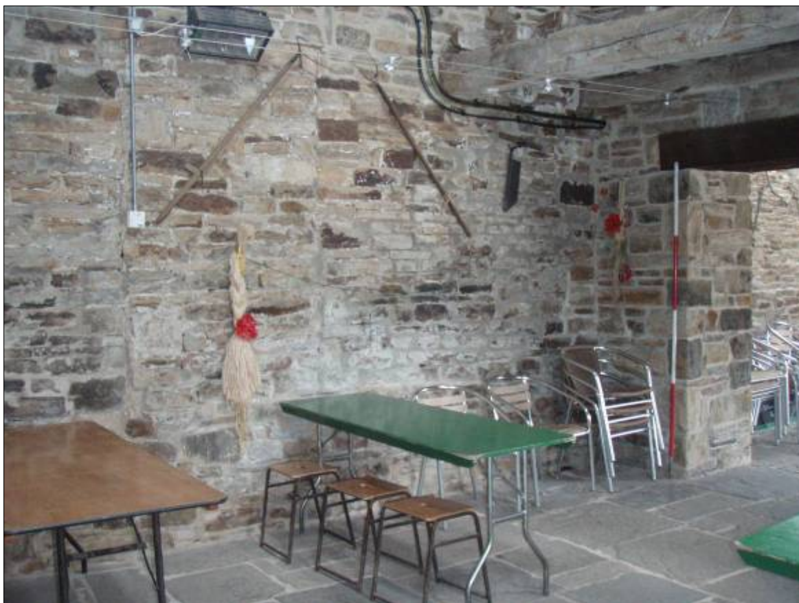
Plate 38. Interior of Building I facing northeast, showing scar of a cruck blade in the northeast corner.
