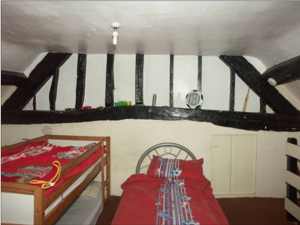
Plate 25. Attic Level of Building F. Interior north side of partition with reused tie-beam.
