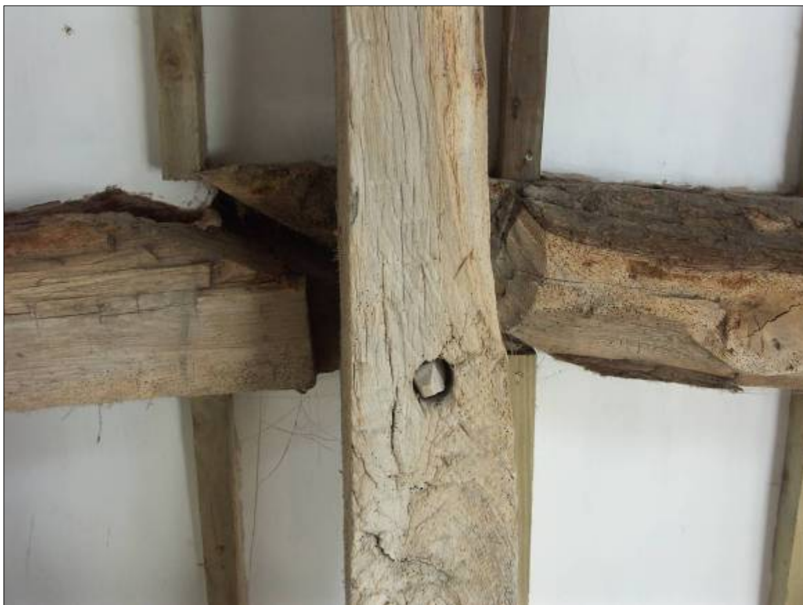
Plate 44. Detail of the joint for the side purlins in the surviving cruck frame
