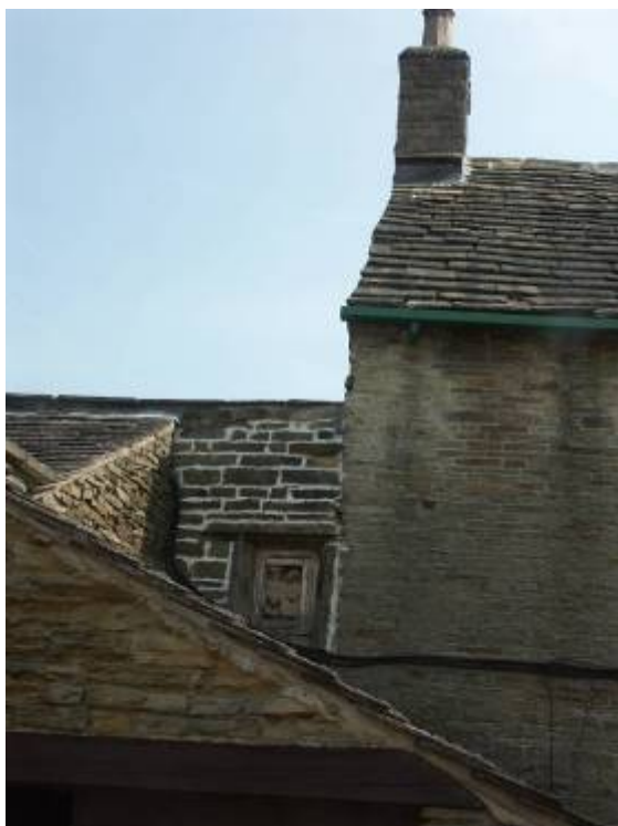
Plate 15. Junction of Building F and Building G, showing the ragged north end of Building F where part of the structure has been demolished.
