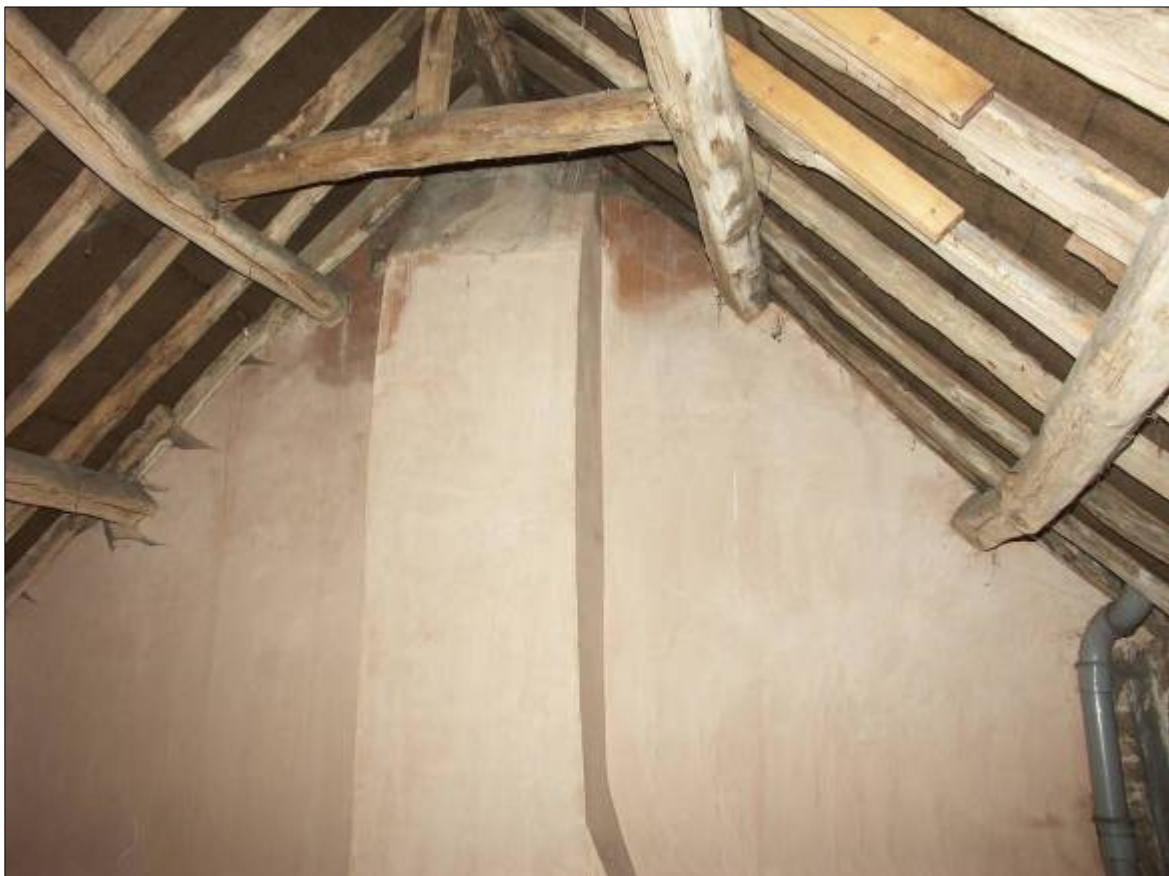
Plate 22. Attic level of Building F. Interior showing the inserted chimney flue in the south wall.
