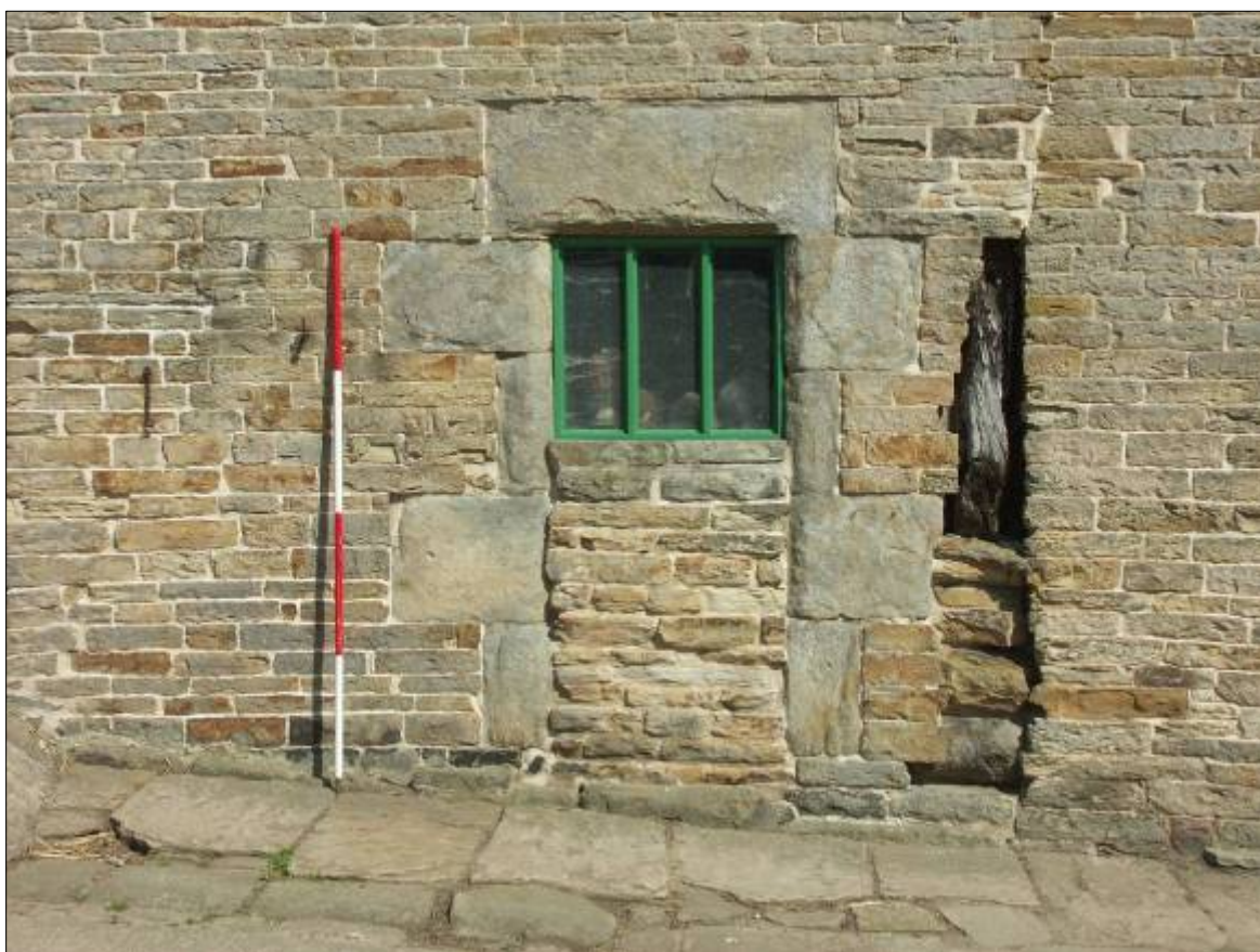
Plate 37. Detail of exposed cruck blade and stylobate beside a partially blocked doorway in the south wall of Building I.
