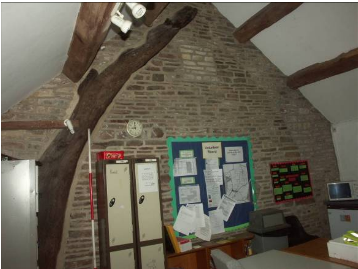
Plate 73. First Floor of Building O. Interior of the south wall showing surviving cruck blade and the scar of its matching pair.
