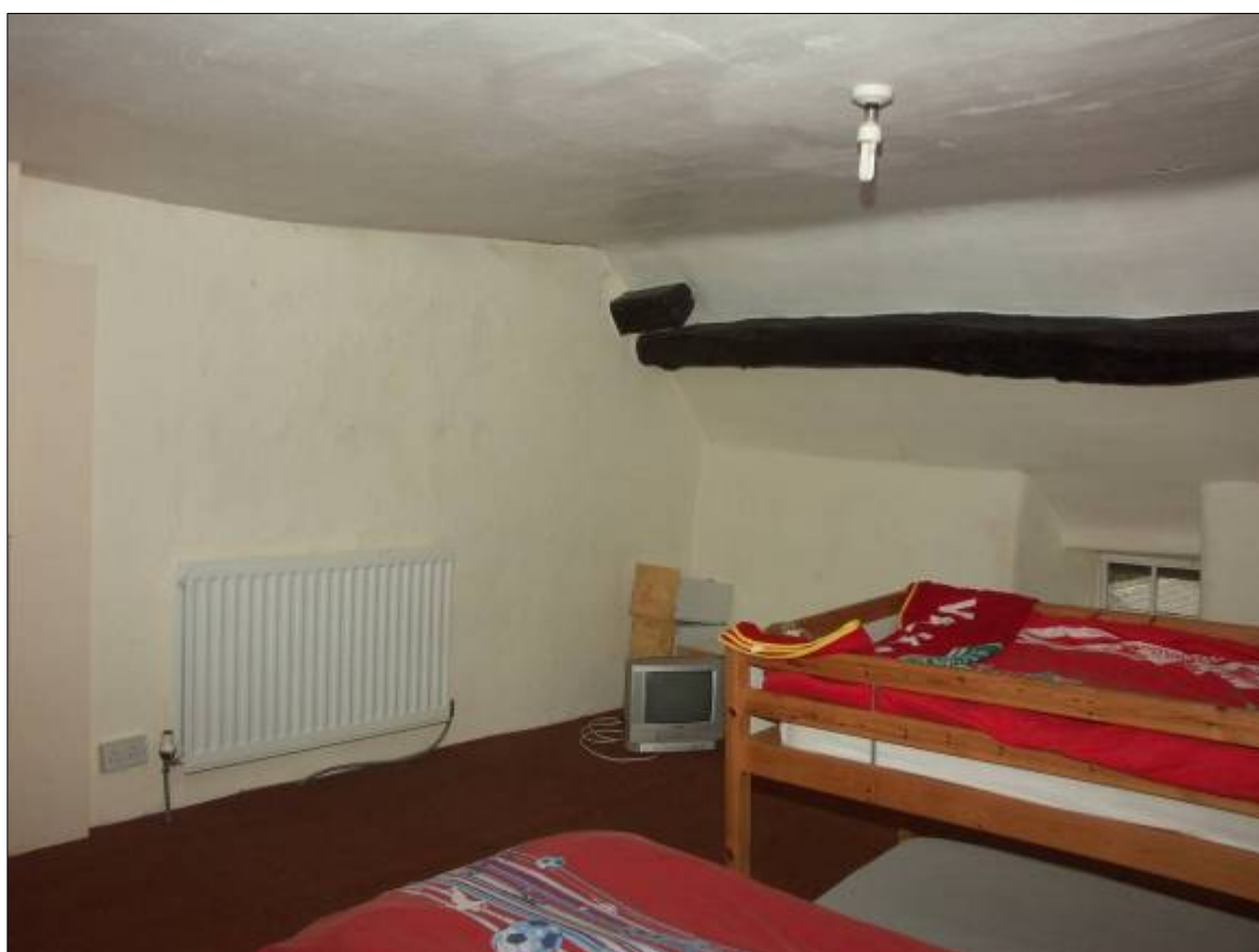
Plate 20. Attic Level of Building F. Interior north wall showing side purlin leading to the now demolished northern half of the building.
