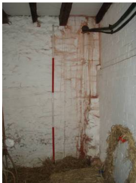
Plate 40. Interior of the western half of Building I showing the scar of a cruck blade in the northwest corner.
