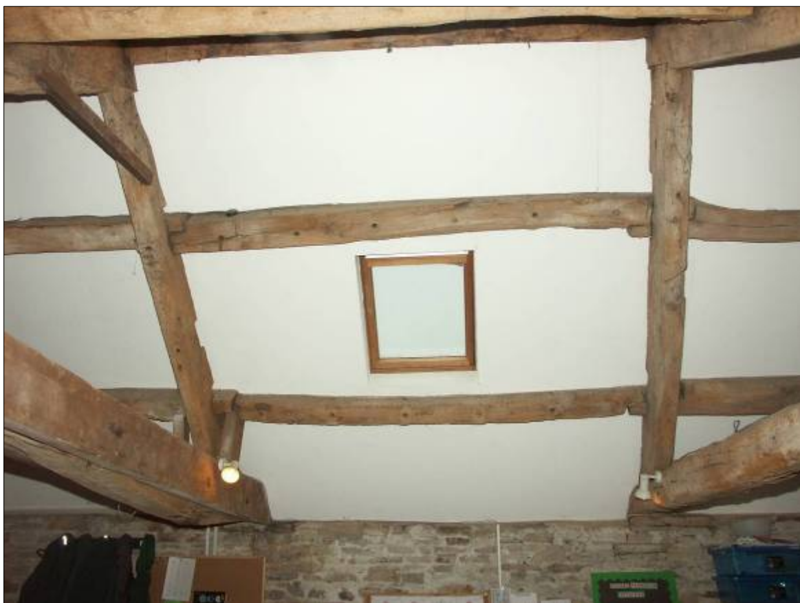
Plate 77. First floor of Building O facing west showing reused timbers with auger holes used as the side purlins.
