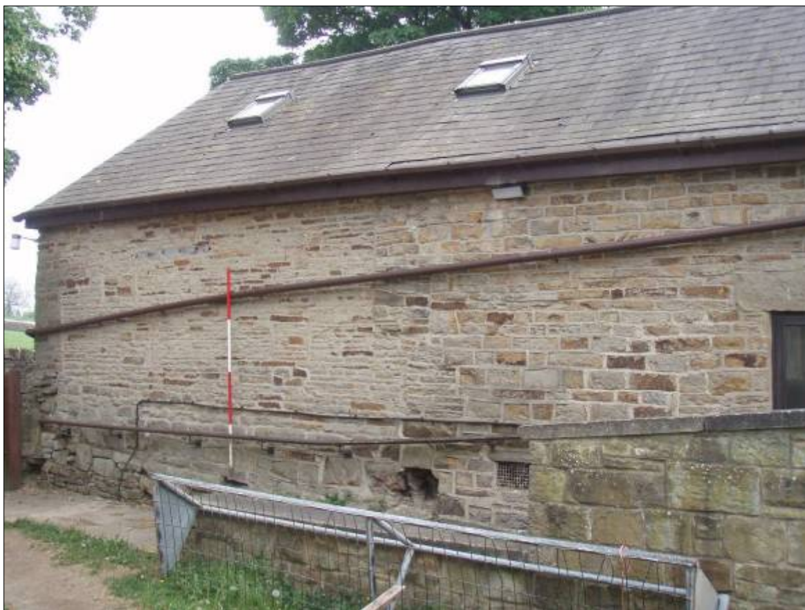
Plate 70. North portion of the west elevation of Building O showing blocked features associated with a demolished building running east/west
