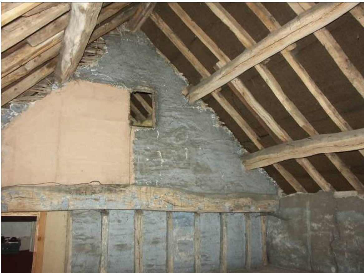
Plate 24. Attic Level of Building F. Interior south side of partition wall with reused tie-beam.
