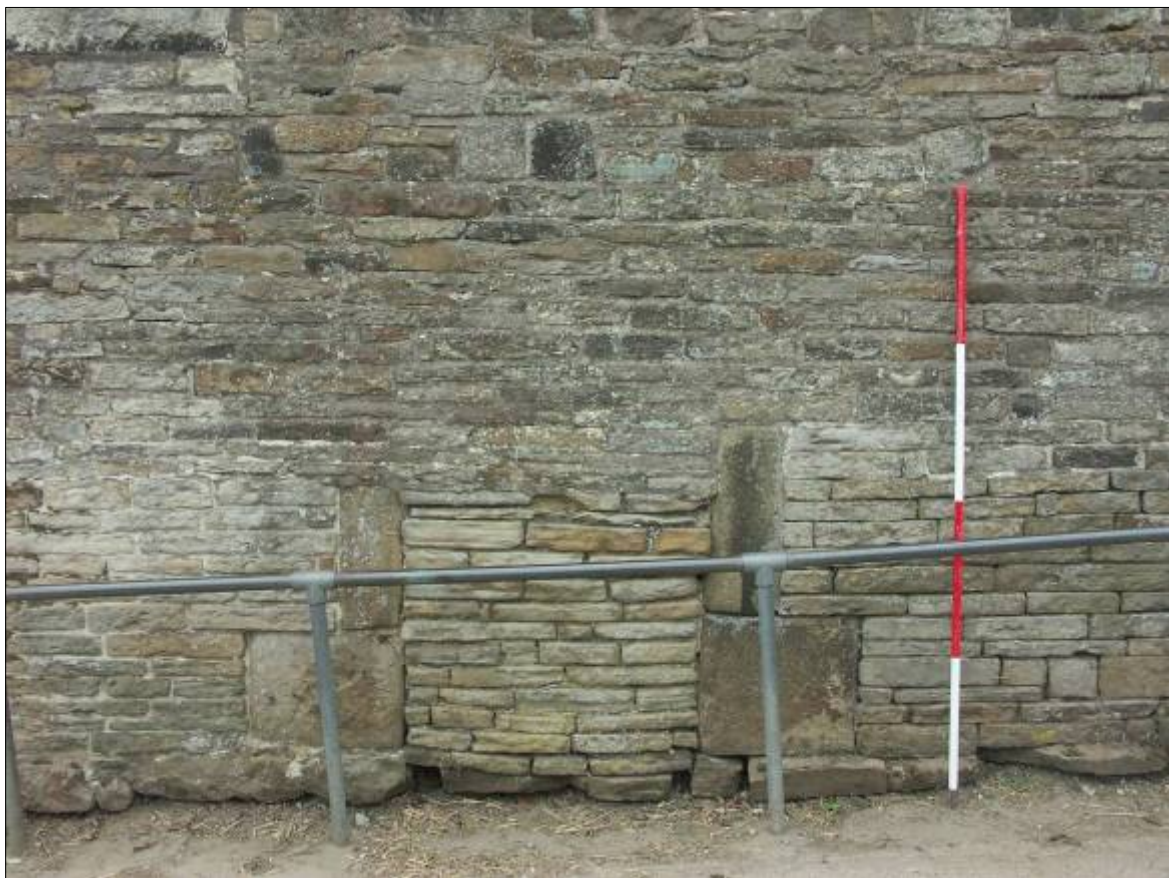
Plate 18. Detail of blocked and truncated doorway in the north wall of Building G.
