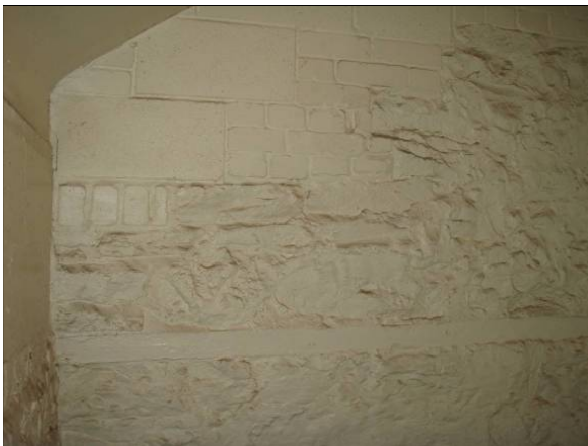
Plate 93. First Floor of Building S. Interior showing modern brick and concrete heightening of the side walls and gable end. The slender tie-beam of a previous roof structure is also visible embedded in the wall.
